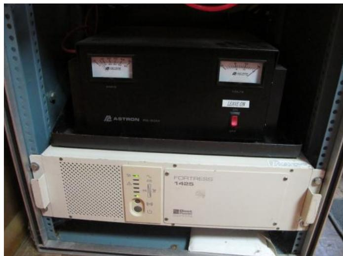
does not supply power for things such as the linear amplifiers. Also one should be careful not to plug in anything like an electric heater to an outlet marked UPS. It uses four 7ah batteries.
